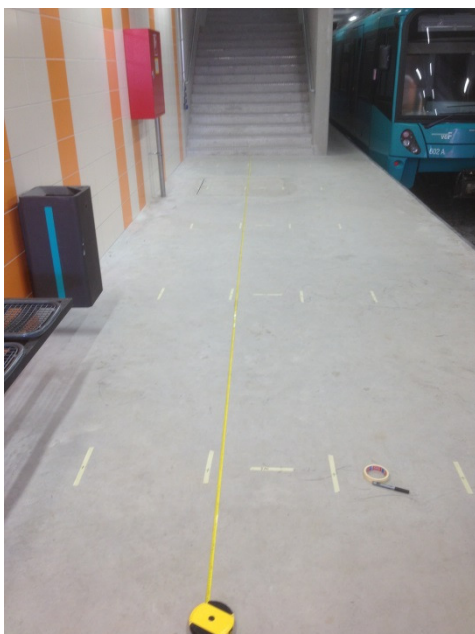
Figure 3.12 The possible positions of the fans are measured, marked with tape and the distances are written down on the tape.
