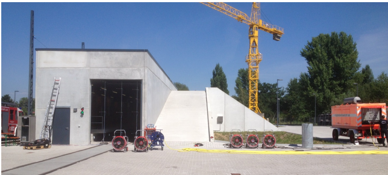
Figure 3.8 The summary of all the materials used during the tests. The underground building is in the background. The five fans are in the middle. The 156 kVA generator is on the right. It is connected to the fans by means of several cables and a distributor cabinet (64A→2x32A). The cabinet with the pressure transducers, voltmeters, and laptop is on the left. The bidirectional probes are positioned in the entry opening for the underground trains.
