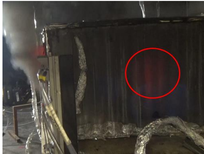
Figure 13: Hot spot on the compartment walls for the closed ceiling case
