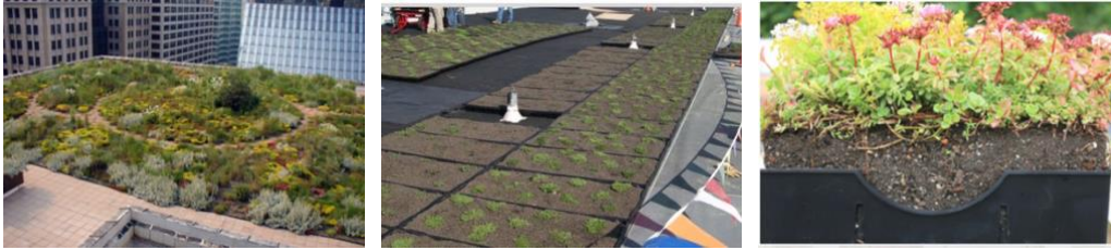
Figure 8. Green Roof Installation Typology Built-In-Place System (left), Modular System (center), and Hybrid System (right) Sources: FM Global Loss Prevention Data Sheet 1-35 & Green Roof Design [24] & [25]
