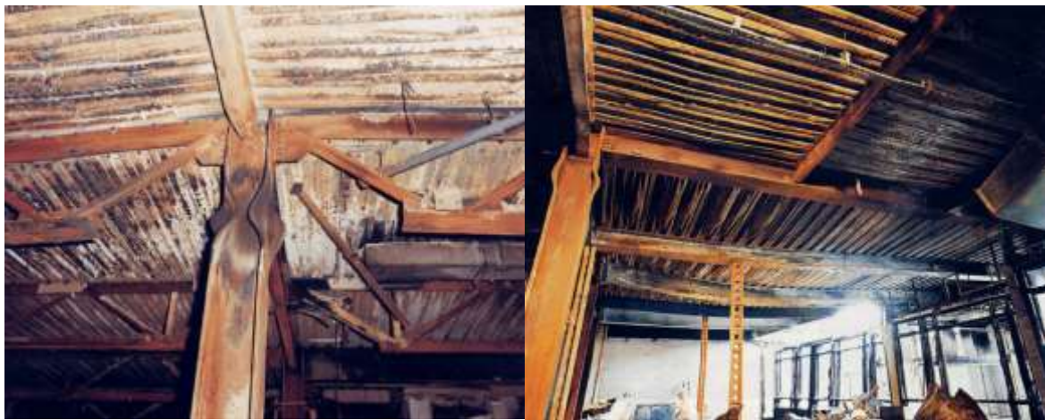
Figure 12. Local buckling of columns. Extracted from P112 Investigation of Broadgate Phase 8 Fire [4].
