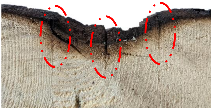
Figure 30. Second cut of the first test showing signs of delamination
