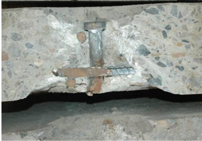
Fig. 19 : Headed stud shear failure at 200°C (Mirza, Uy and Krezo, 2011)
