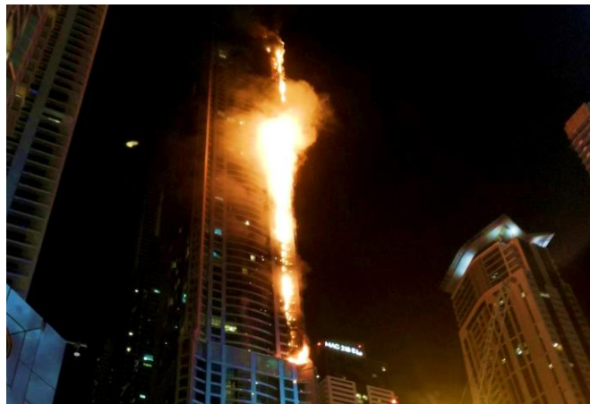
Figure 36 Torch tower fire, Dubai
