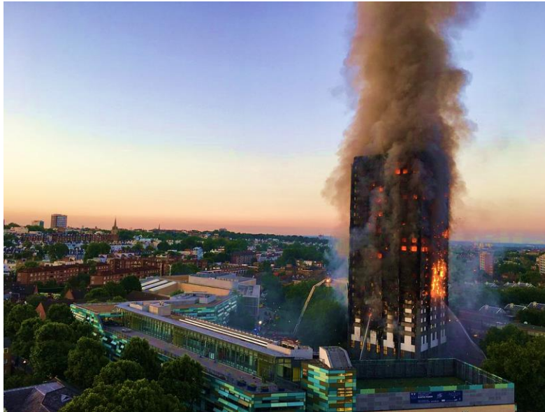
Figure 37 Grenfell tower fire, London
