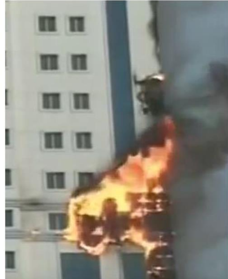
Figure 3 Rotational fire spread observed in a building fire (Taken from Peacock et al., n.d.)
