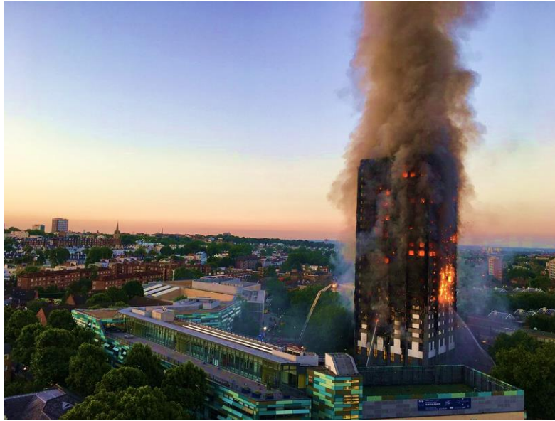
Figure 37 Grenfell tower fire, London
